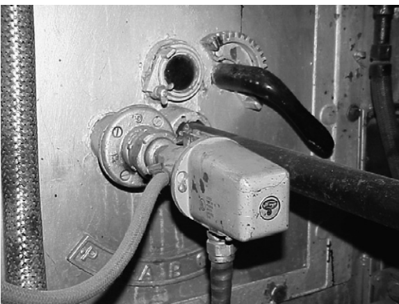
Exhibit 3. Typical optical flame detector that monitors flame conditions.
